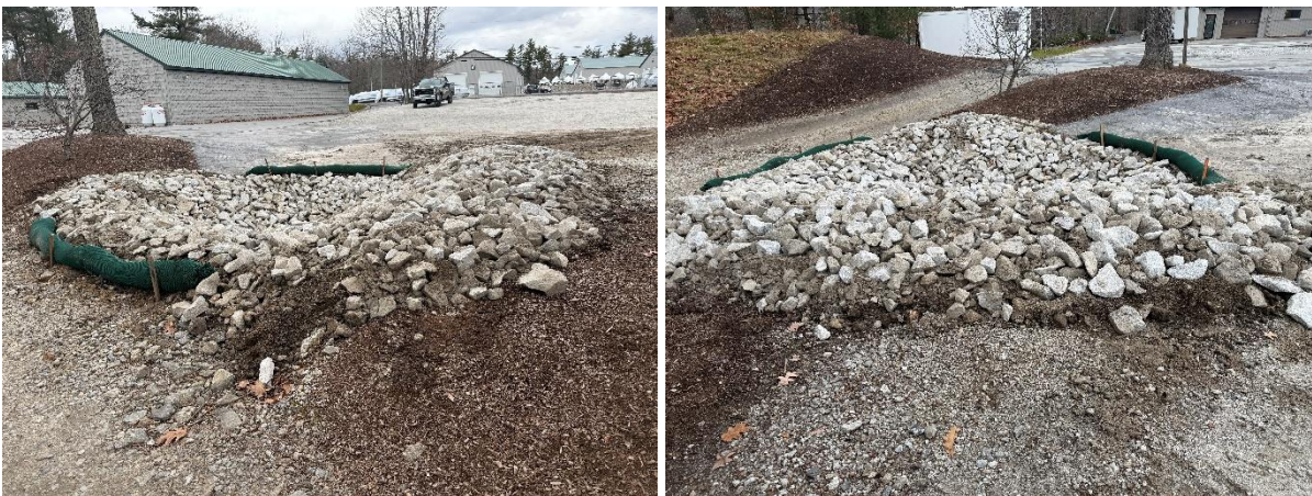
Photos of the improved retention basin, deeper, lined with rip rap, and stabilized with coir logs. Photos provided by MacCallum's Boathouse.
