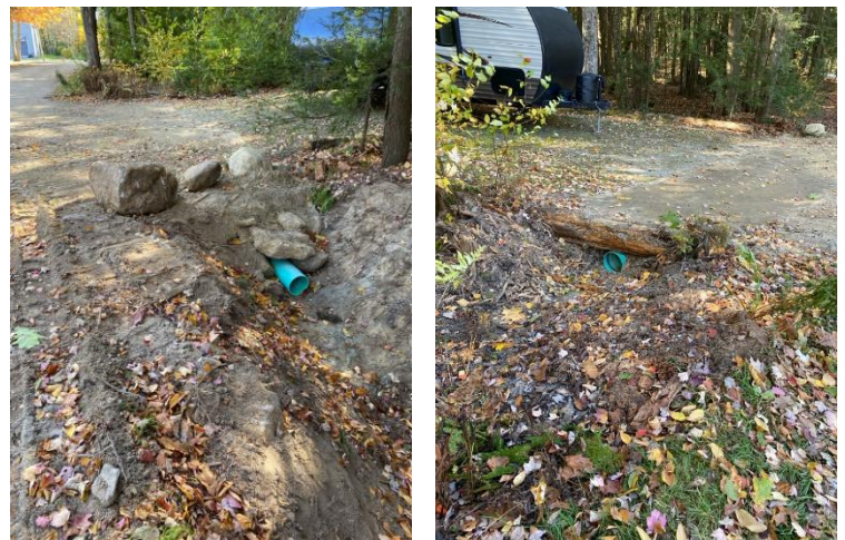
Eastern (left) and western (right) views of the small infiltration area.
