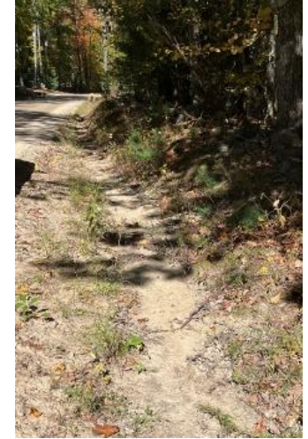
(Left) Three pipes appear to route water from a nearby home to the culvert inlet. (Right) Road shoulder ditch erosion at the site.
