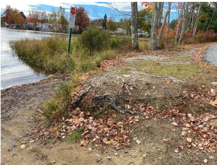
(Left) Exposed roots and a steep drop off of the shoreline to the water's edge indicating erosion, (right) the end of the paved boat ramp where it meets the water.
