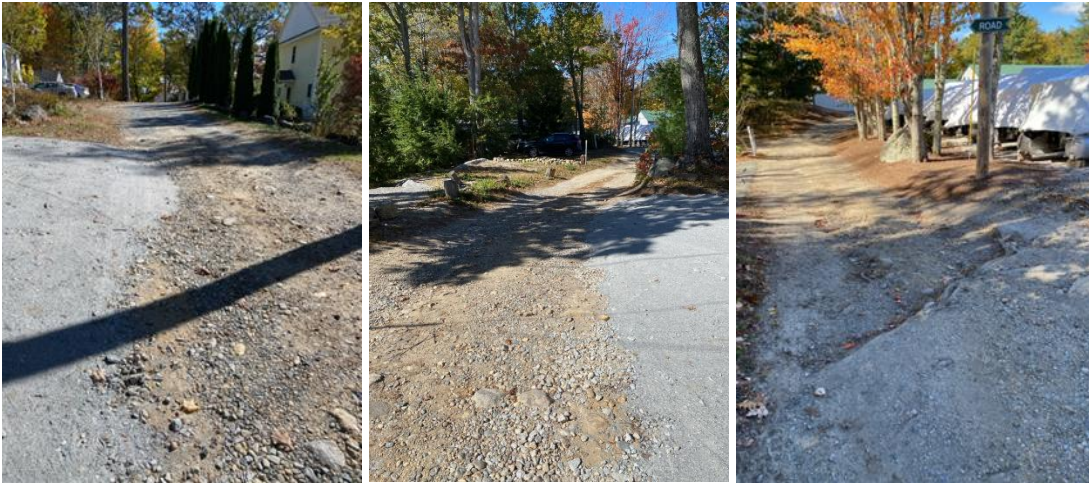
(Left) Lake Road facing east, (middle) west, (right) and behind the boat yard.
