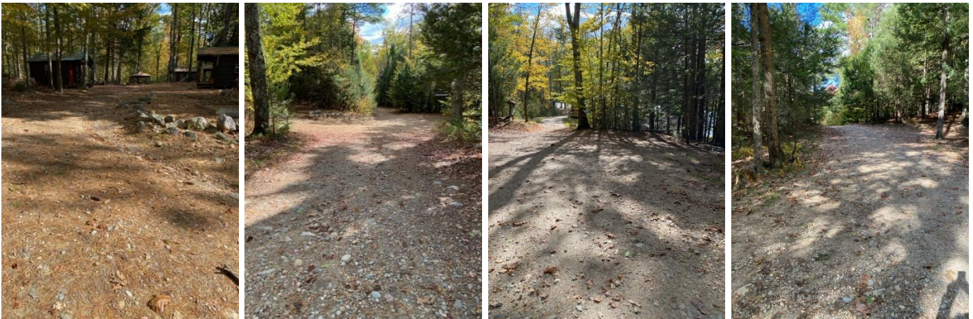
(1) Stormwater flow path coming from the cluster of cabins to the primary camp roadway (2). (3 and 4) Two of the three areas along the roadway where it widens and the infiltration basins could be created, minding snow maintenance needs.
