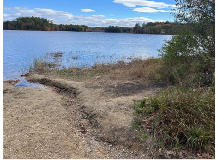
(Right) The steeply sloped paved area directs stormwater to the lake. (Left) A large gully has formed at the bottom of the boat launch.
