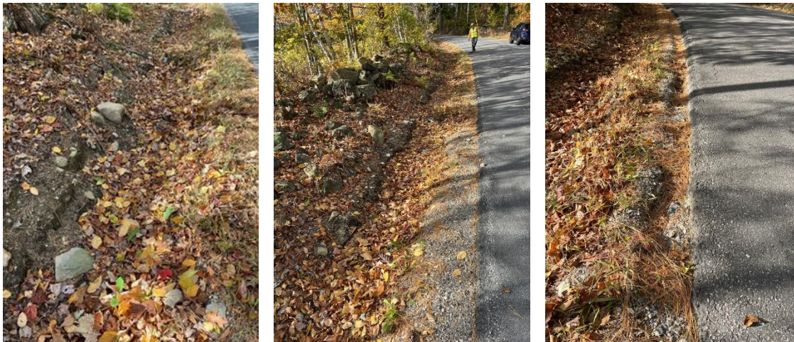
(Left & Middle) A well-defined gully is present in the road shoulder ditch, which is typically bare, but was filled with fallen leaves at the time of the survey. (Right) The road shoulder of Harmony Road is eroding into the ditch.
