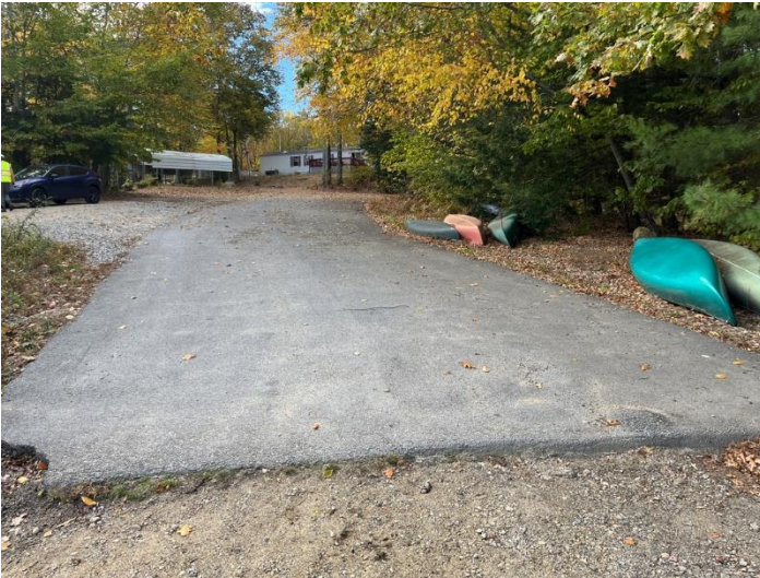
(Right) The steeply sloped paved area directs stormwater to the lake. (Left) A large gully has formed at the bottom of the boat launch.
