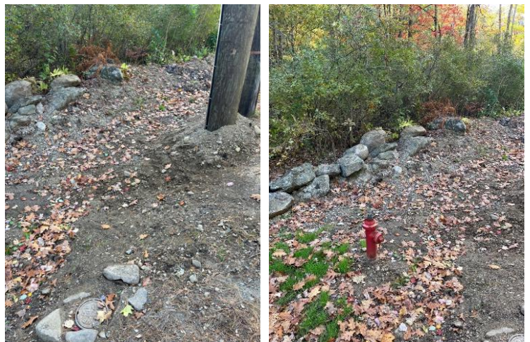
Bare soil areas in the road shoulder ditch.
