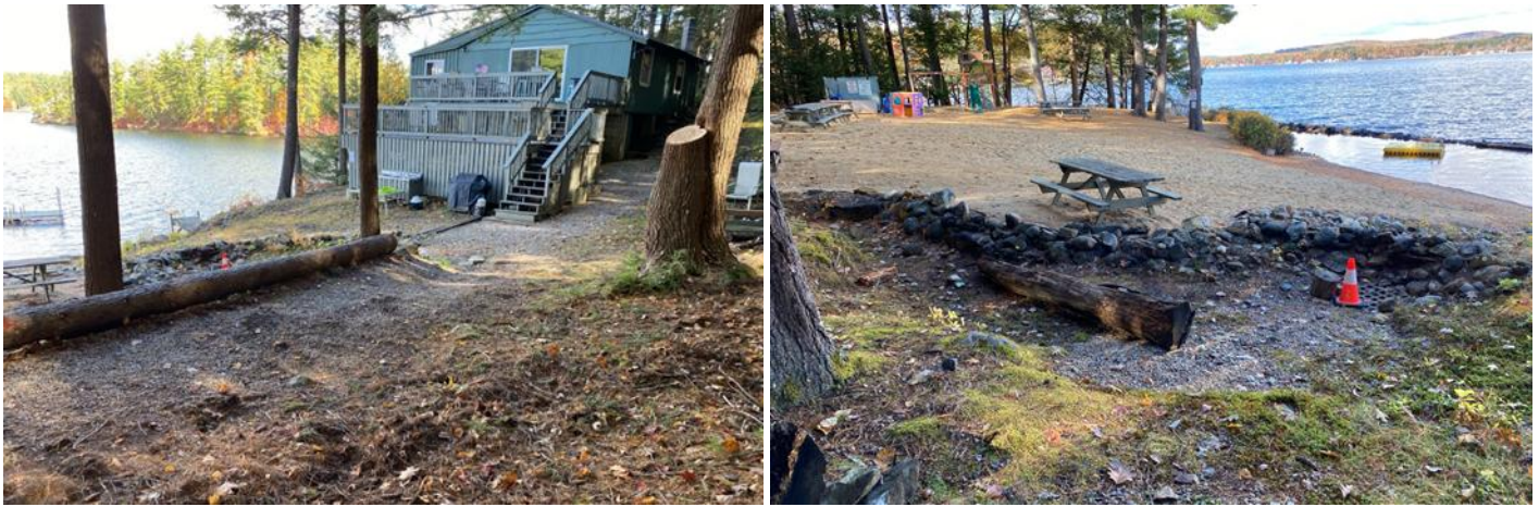
(Left) a walkway leading to the club house with a tree trunk for stabilization. (Right) The last retention basin with the outflow grate next to the orange cone.
