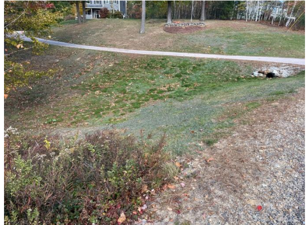
Stormwater exits the under-driveway culvert and enters the stream after traveling through a sloped, grassed area.
