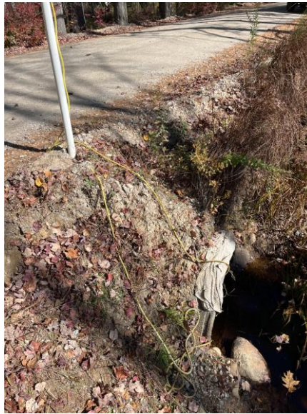
(Left) The streambank at the culvert outlet is eroding, partly due to a crumbling berm. (Right) The stream is part of a larger wetland complex.
