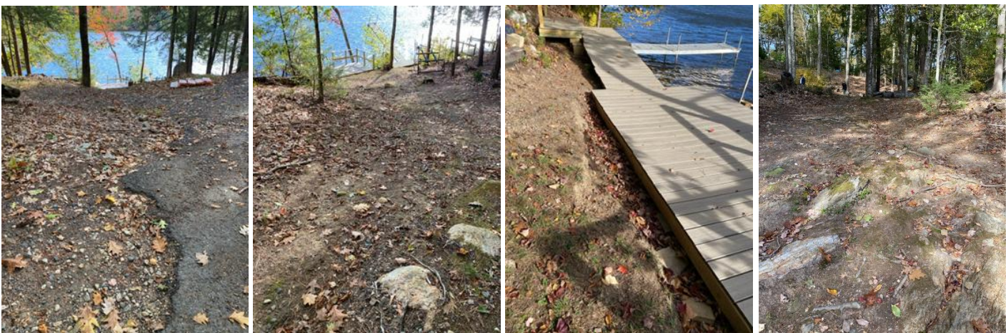
(Lef two) Lagoon Road slopes steeply to the side towards the lake. (Right two) Gullies lead to the dock along the water.
