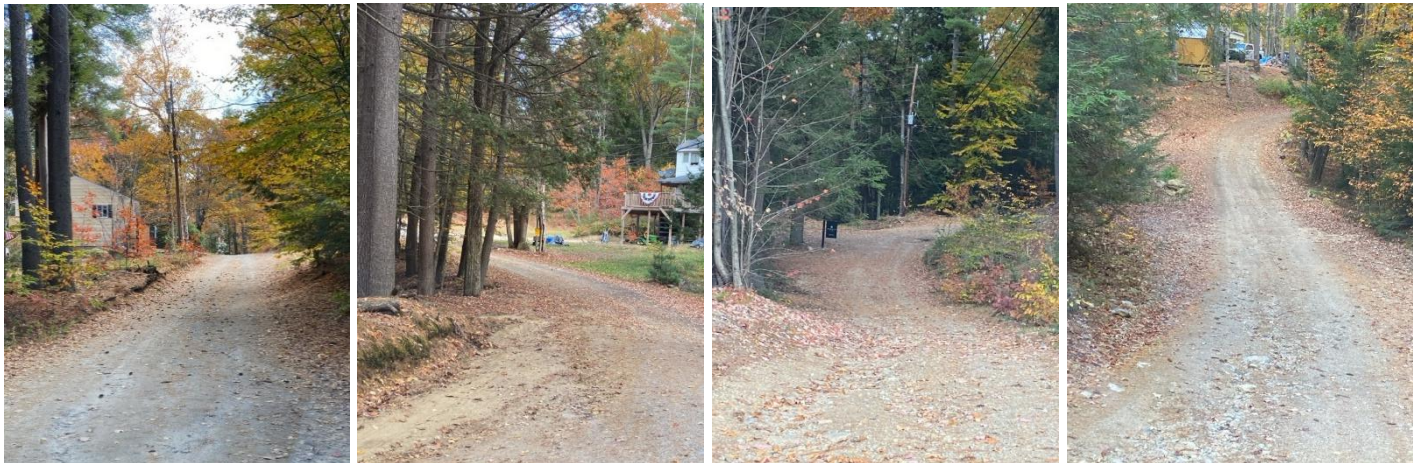
Erosion gullies and stormwater flow paths on the road surfaces of Rita's Circle and Jack Street.
