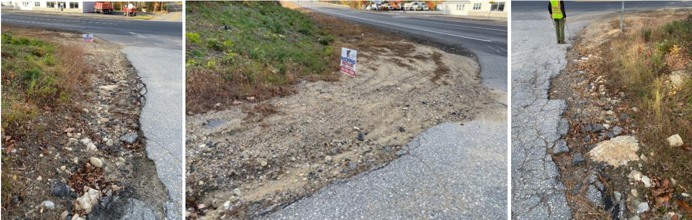
Western road shoulder (left and right), and eastern road shoulder (right).
