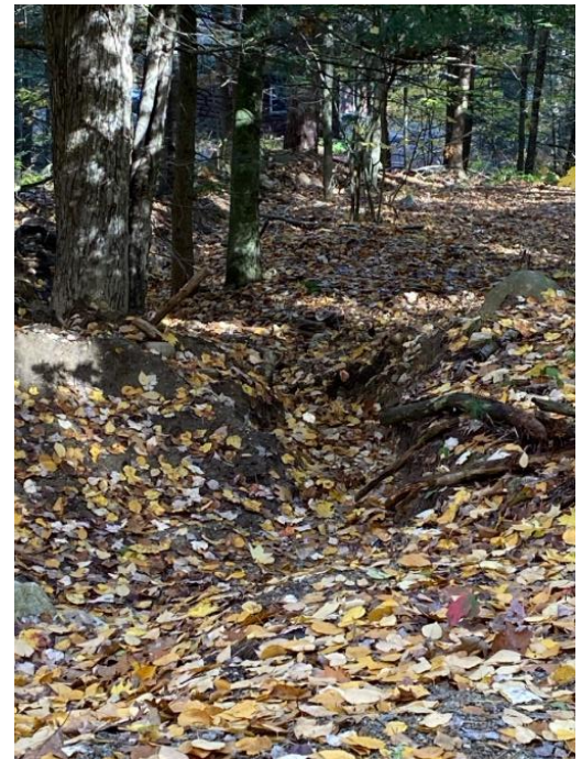
The downhill view of the ditch/flow path with caving edges and exposed roots.
