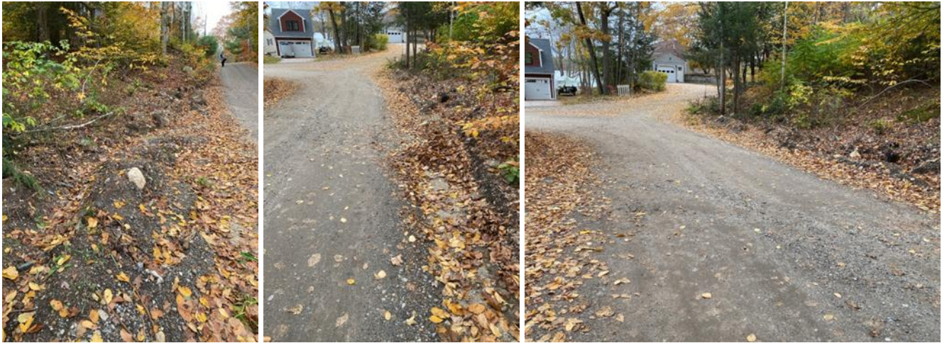
(Left) Southern road shoulder gully looking uphill. (Middle) Southern road shoulder gully looking downhill. (Right) Flow path of the road shoulder flow crossing Birch Street to the intersection with Shore Drive.
