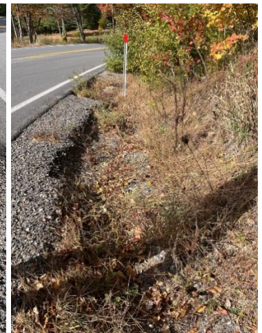
Road shoulder erosion on Catamount Road. Eroded material enters a catch basin designed for high stormwater velocities.
