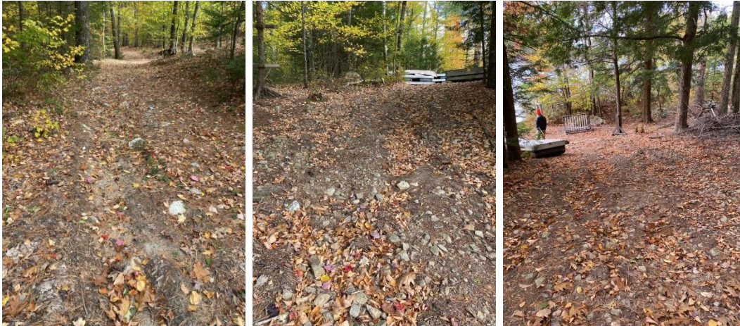
(Left) Camp road with gully, (center and right) camp road as it slopes down to the water from the dock storage area.
