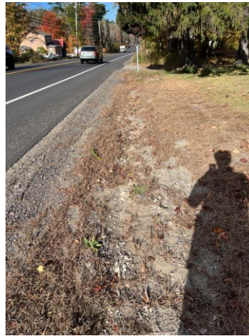
(Left) Road shoulder erosion leading to a catch basin.
