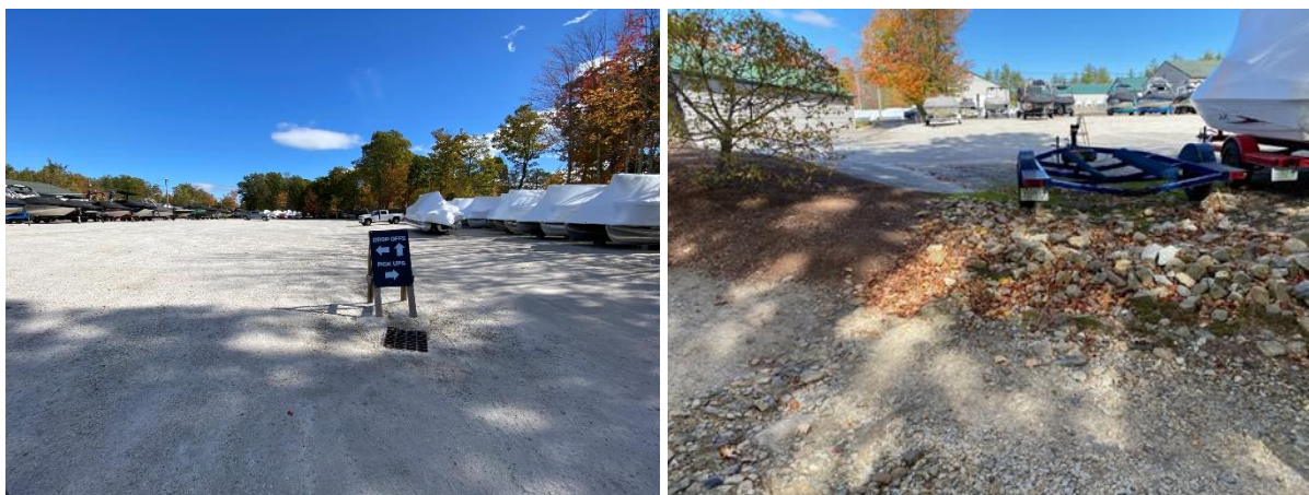
The boat yard catch basin (left) and the original retention basin and breakthrough path during the watershed survey (right).
