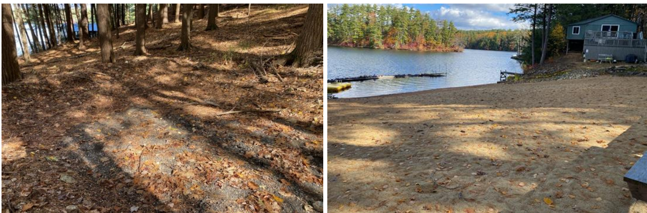
(Left) The first retention basin with lots of accumulated road surface material. (Right) No large erosion gullies were observed across the beach area.
