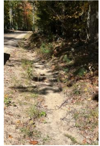
(Left) Three pipes appear to route water from a nearby home to the culvert inlet. (Right) Road shoulder ditch erosion at the site.
