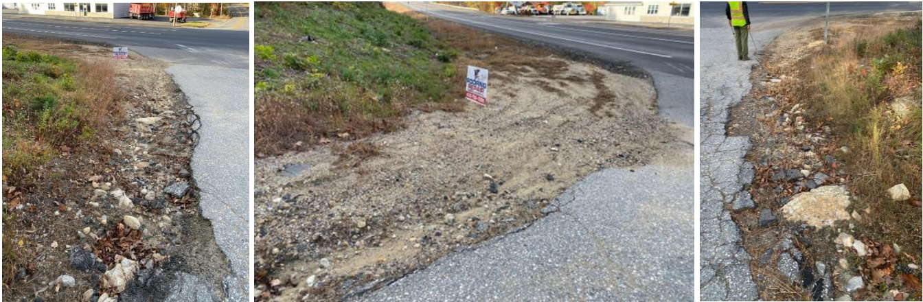
Western road shoulder (left and right), and eastern road shoulder (right).
