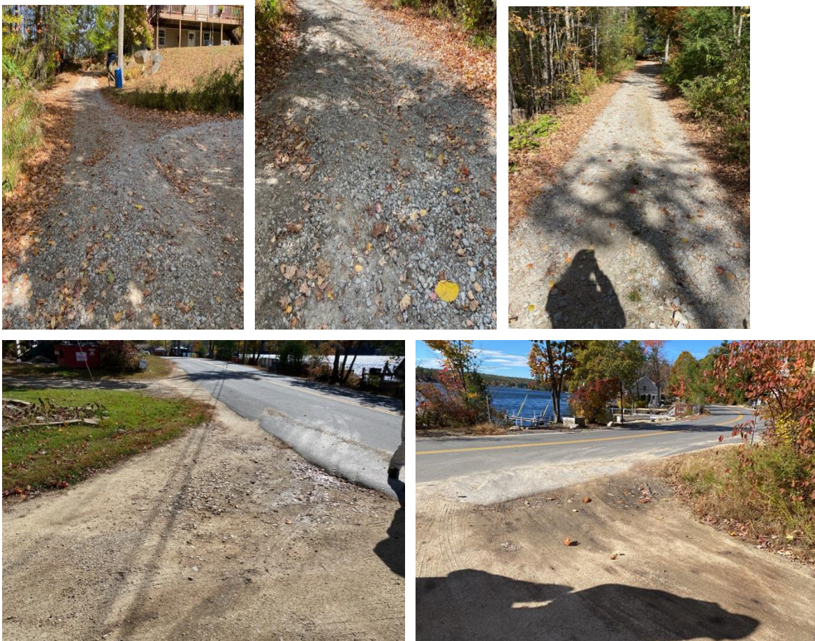
Photos of Wildwood Ave from the intersection with Maple Ave to the intersection with Lakeshore Dr. (paved).
