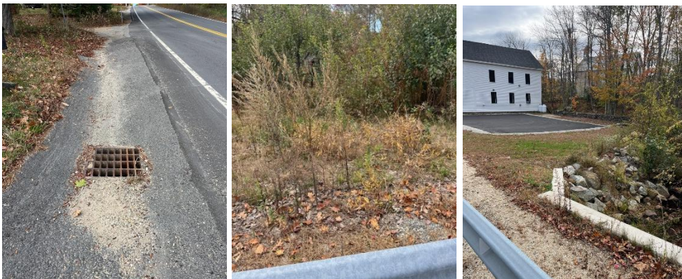
(Left) Sediment from the road enters the catch basin through the paved swale. (Middle & Right) Vegetated areas that may be used to infiltrate stormwater.
