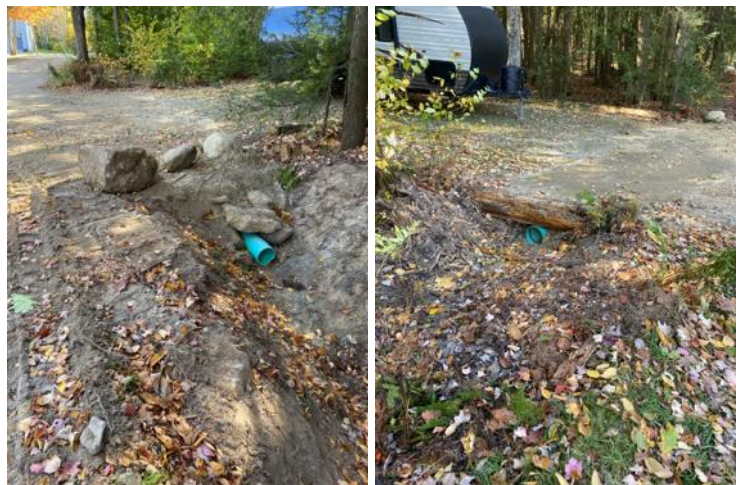
Eastern (left) and western (right) views of the small infiltration area.
