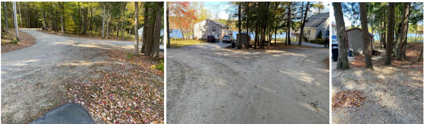
(Left) Sleepy Hollow Road intersection looking up the roadway where it splits to access shoreline properties. (Middle) Sleepy Hollow Road intersection looking downhill, towards Northwood Lake. (Right) Stormwater flows through the patch of pine trees behind the little shed.
