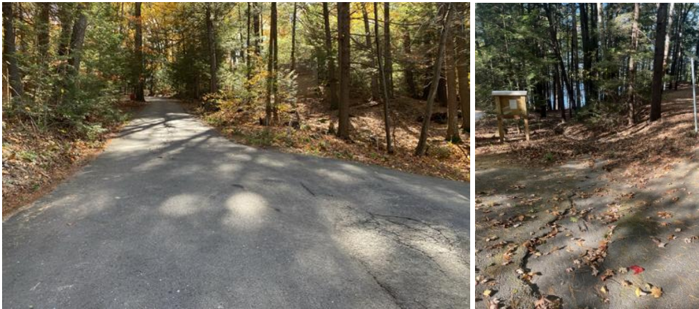
(Left) View up Cole Road with the paved swale in the bottom right corner, (right) the paved swale entering the forest.
