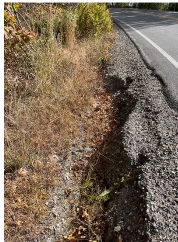
Road shoulder erosion on Catamount Road. Eroded material enters a catch basin designed for high stormwater velocities.
