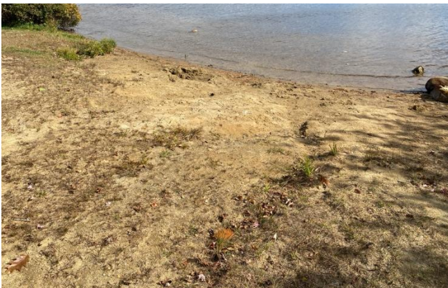
Erosion gullies were observed between the beach area and the water's edge.
