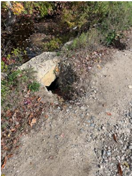
(Left) Severe erosion at the culvert outlet. (Middle) View of twin culverts. (Right) There is minor erosion at the culvert inlet.
